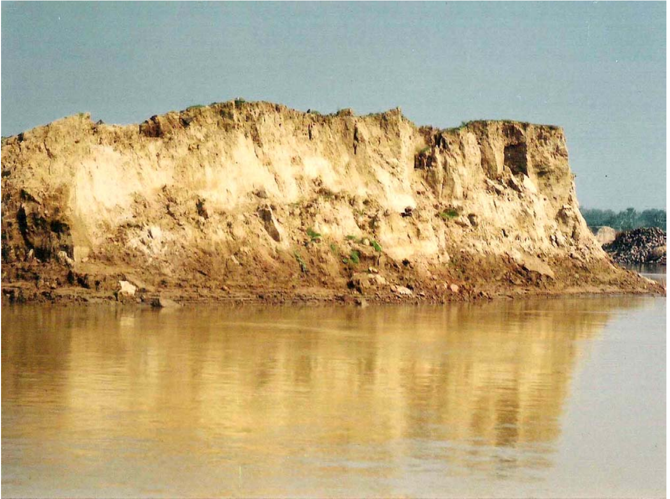
Plate-6: The relic of Embankment no.8 stands on the river (September,2004).
