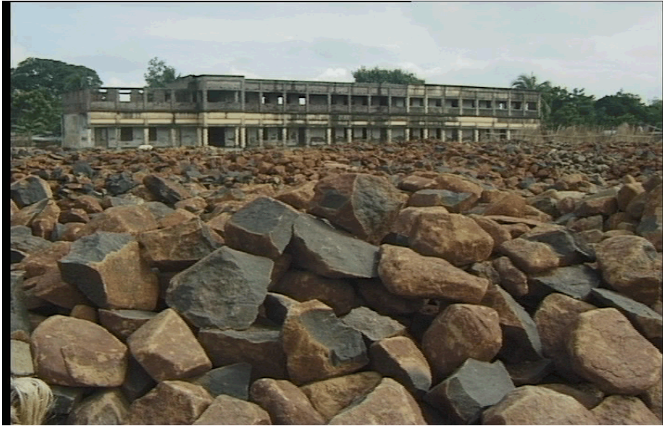
Plate-7: Akheriganj(2000)- the boulders did not ensure protection against erosion.
