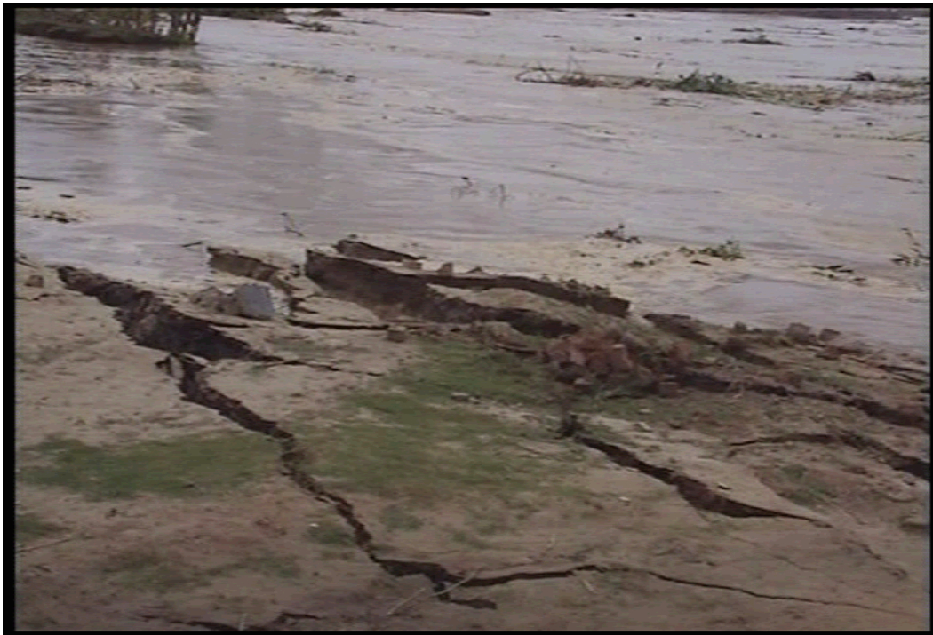
Plate-3: Linear cracks developed along the bank due to undercutting of basal sand-layer.
